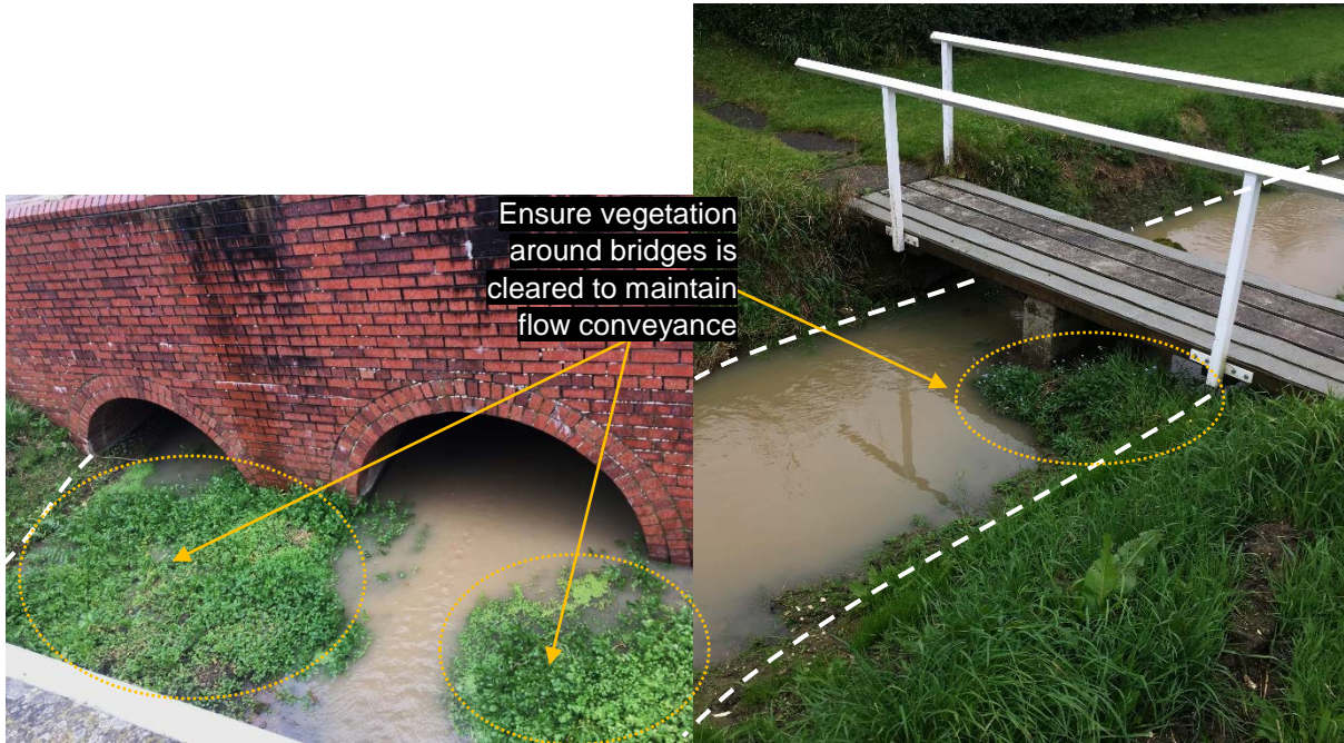
Figure 5: Special attention should be paid to in-channel structures such as bridges to ensure flow is not restricted around them. These images show examples of vegetation for removal. Operatives will not enter any confined space to achieve this as a part of this work.
