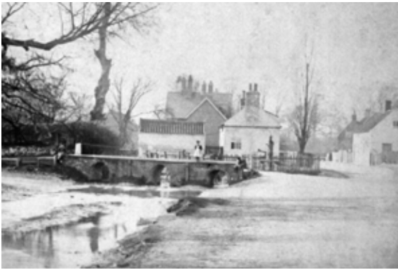
High Bridge pump.
