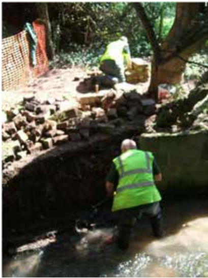
2010. Opening the cascade constrictions to prevent further flooding.
