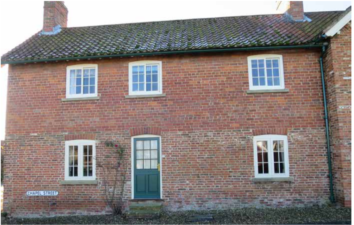
The Old Forge on the corner of Thorpe and Chapel Street is another example of adding a second storey with wider bricks.
