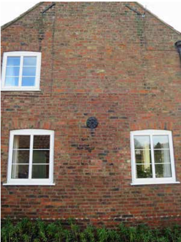
Although the date plate of 70 Front Street suggests that the house was built in 1885 in fact the lower part dates from 1772 as can be seen from the change in bricks. Mr R L Wardell added the upper storey later.
