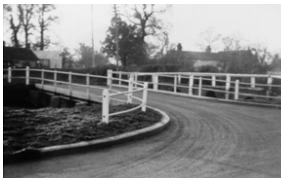
This road bridge replaced the ford in the 1950s. It was later deemed too weak to support the traffic using it so a new bridge was built of 16,000 red bricks in 1995.
