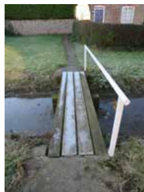
1924 Mrs Hudson sent a requisition to have her bridge widened so as to get over it with her pram.
