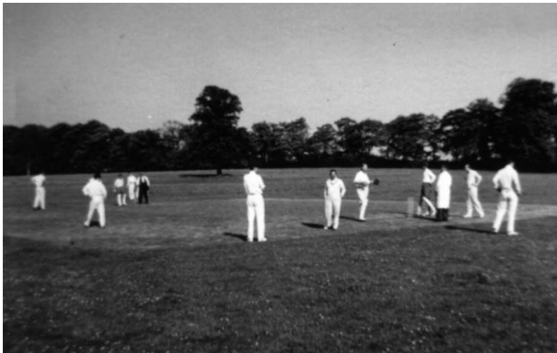
~1960 Cricket on the Marsh. All that remains of the sport is the concrete roller which lies neglected near the Cascade Bridge gate.
