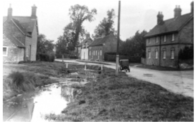
Roads were surfaced with compacted chalk until Tarmac arrived in about 1930.
