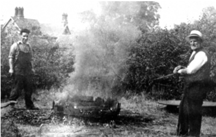
Gordon Miller fitting an iron tyre to a wooden wagon wheel with John Boswell.
