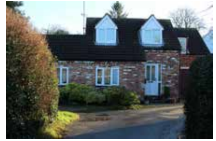
7 Church Lane demolished and replaced in ~ 2000.
