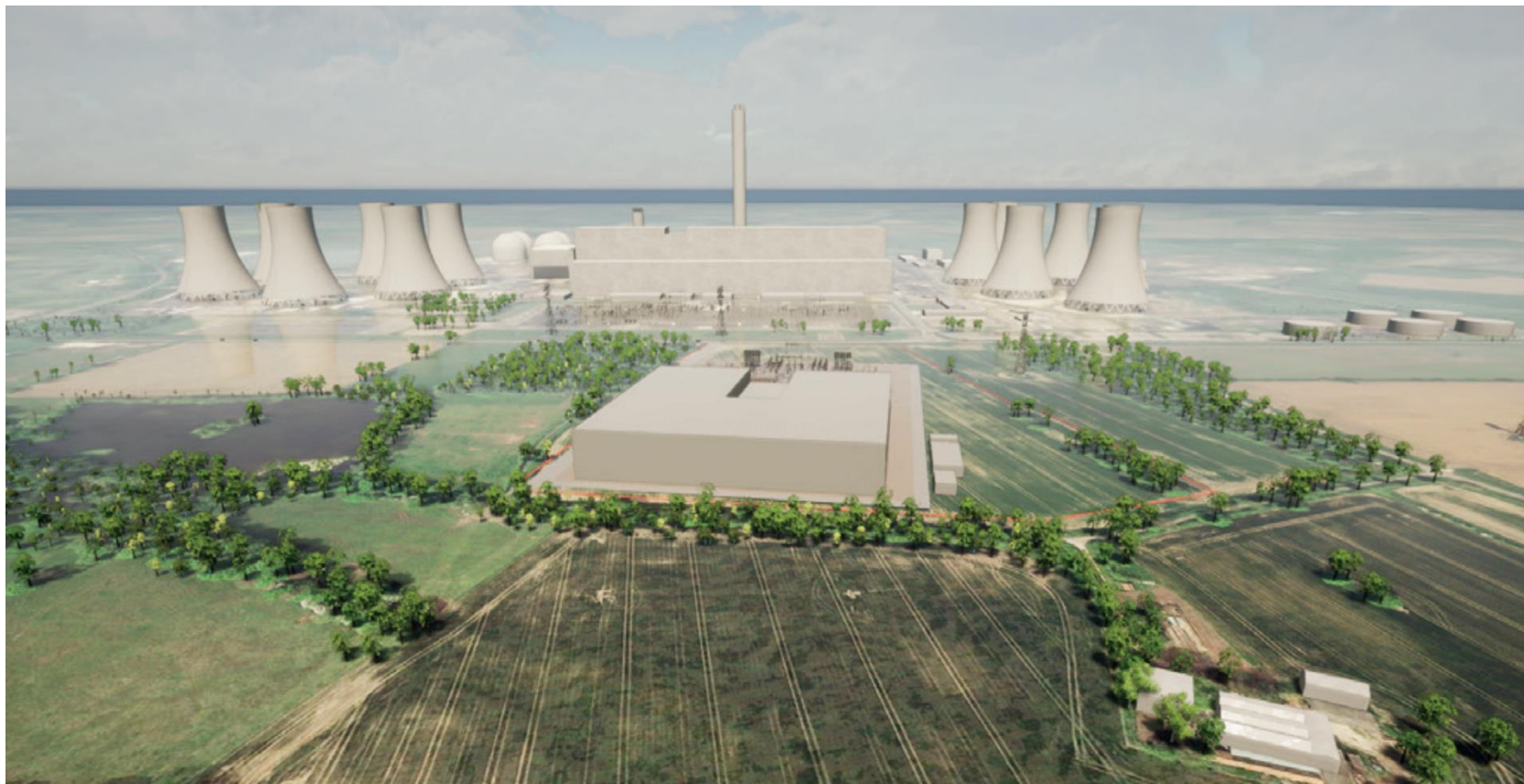
An indicative image of our Drax converter station
